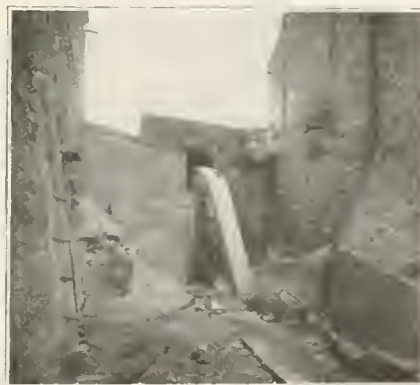
Note the sewer passing under bridges and opening for storm water. House drains enter sewer from either side.
